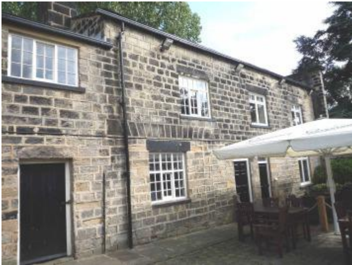
Fig. 8. View of the west side (i.e. from the left) of the building shown in Fig. 7. Photograph taken in the courtyard of the Roundhay Fox.
