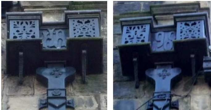
Fig. 9. These Header tanks and fall-pipes used to be at 482, Roundhay Road, currently the Tasty Cafe. They were recently taken down by the owner of the building.
